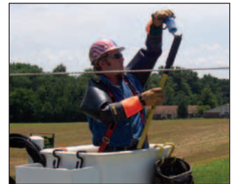
Install the AutoRANGER® with a single hot stick.
