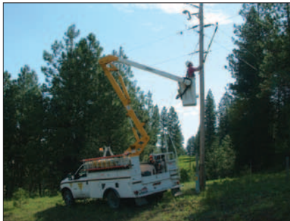
Install the BTRI_IR in applications susceptible to temporary faults.
