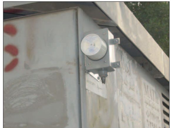
A Ground Fault Detector (Model GFD50SA) provides fault indication in the Middle East.
