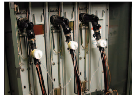
A three-phase Timed Reset Fault Indicator with a remote display (see page 189 for display options).
