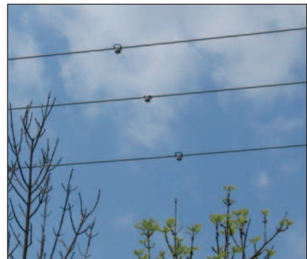
The ERL, SEL's best-selling overhead fault indicator, automatically resets upon system restoration.
