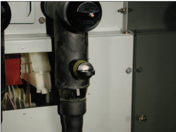
200 A Voltage Indicator alerts utility personnel to the presence of voltage.
