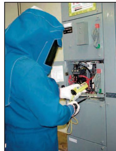
Electrical worker with properly selected personal protective equipment for the hazard.
